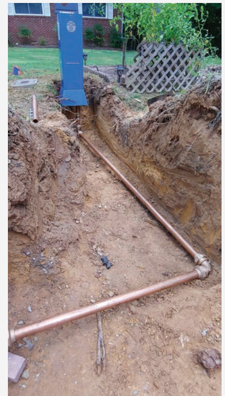
A 2-in. copper pipe connects the station to the water main.
