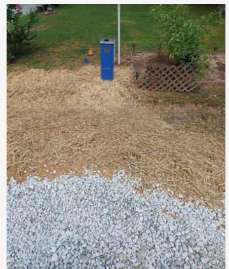
Completed installation of the 3-in-1 Hydro-Guard station.
