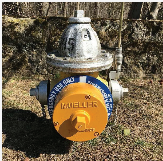
A typical Aquarion hydrant after node installation.
