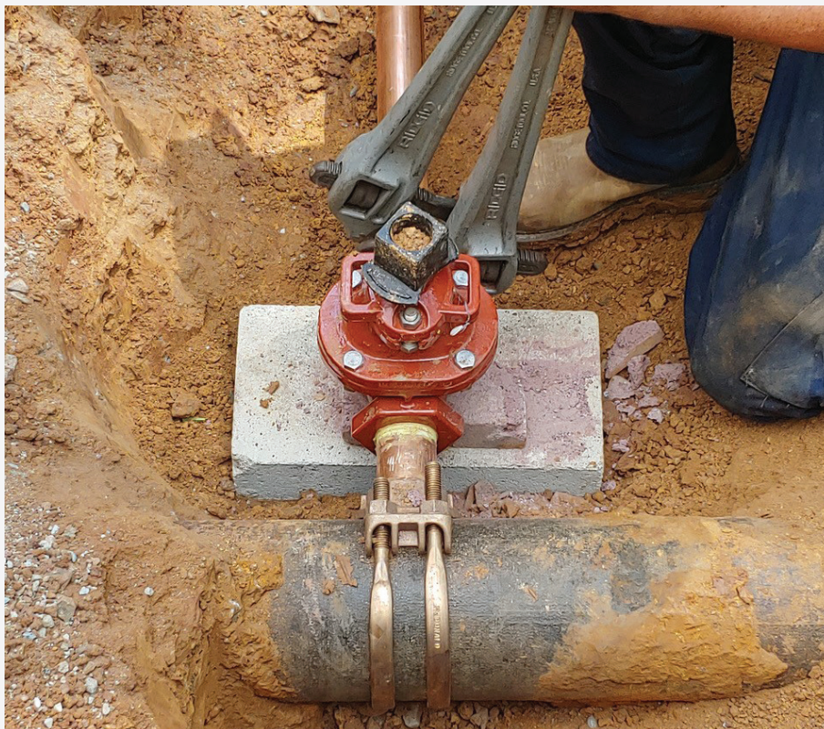
Connecting the 2-in. copper line to valve at the water main.
