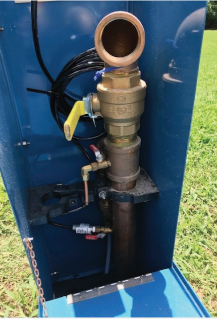
The internal workings of the Hydro-Guard station with remote pressure monitoring, sampling and flushing capabilities.
