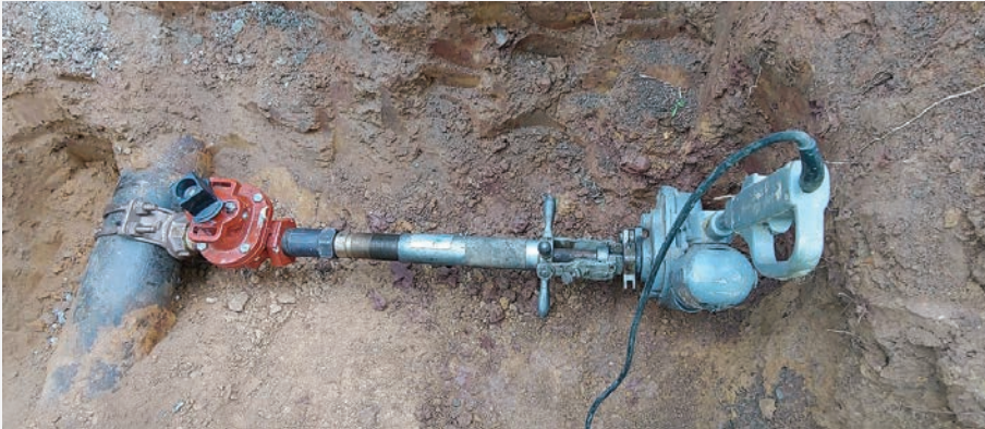
The city's water maintenance staff first added a 2-in. wet tap with a 2-in. gate valve before running a 2-in. copper pipe over to the Hydro-Guard station.
